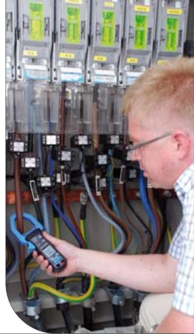
The MD 9230 is a universal current clamp for measuring DC and TRMS AC voltages up to 600 V and DC and TRMS AC currents up to 1000A. With a broad spectrum of measurement functions and features, it is an ideal tool for service companies and works electricians in the industrial sector.
